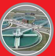
Water Treatment Plant
