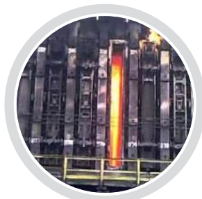
Coke Oven Plant
